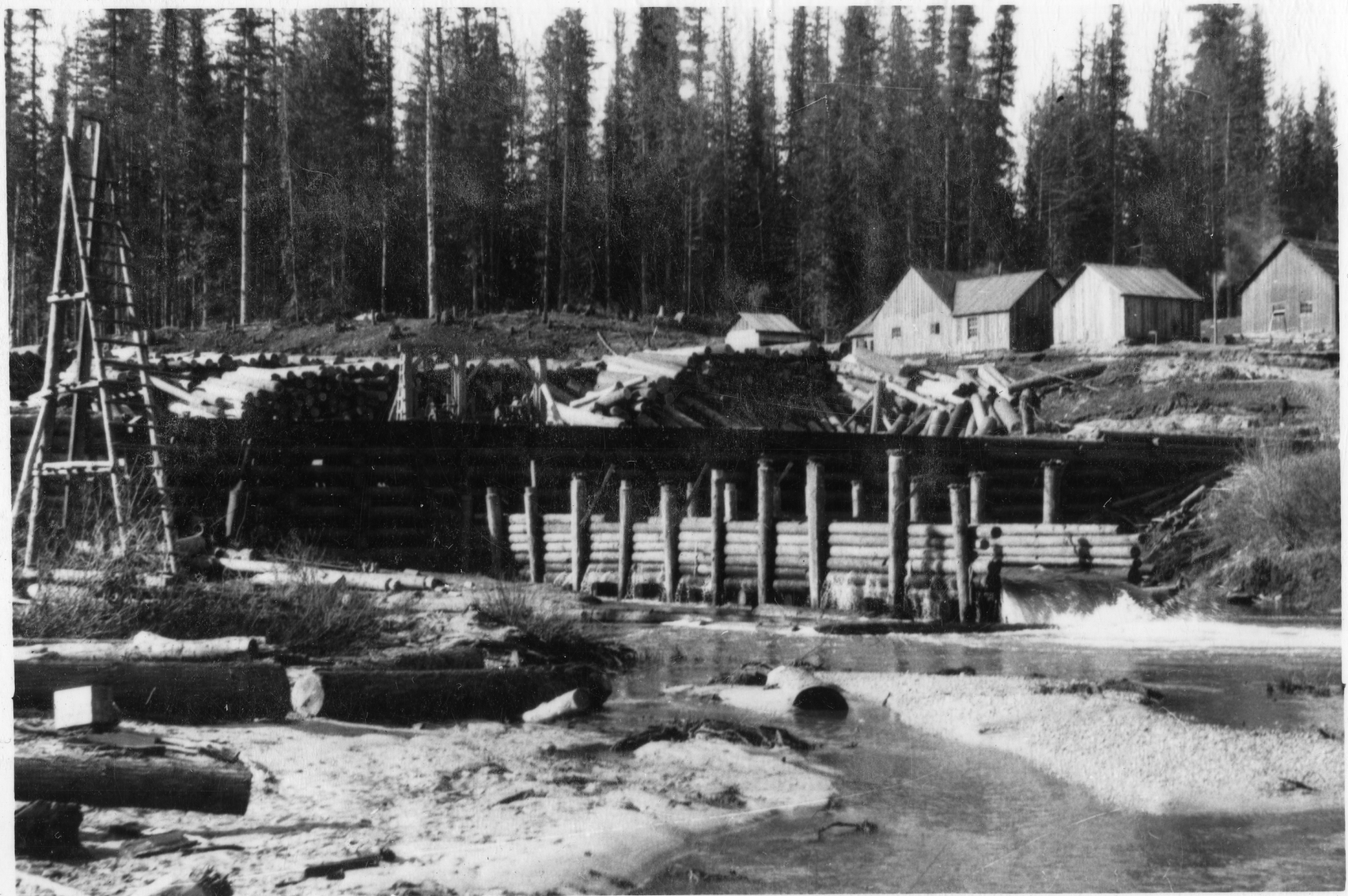
Humbird Dam at camp 19 3/25 (W.G.M)
